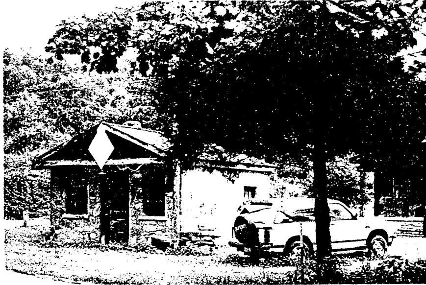
Plate 14. Burgess Store, Looking Northwest.
